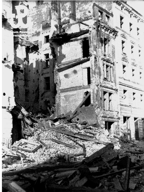
Vertical propagation of the energies of the explosion. (There were big differences in the degrees of destruction of balconies at #1 (only balustrades were blown off) and at #3 (where the whole platforms were gone) - on the right – house at Kilinskiego #3 after bombardment on August 26, 1944.
