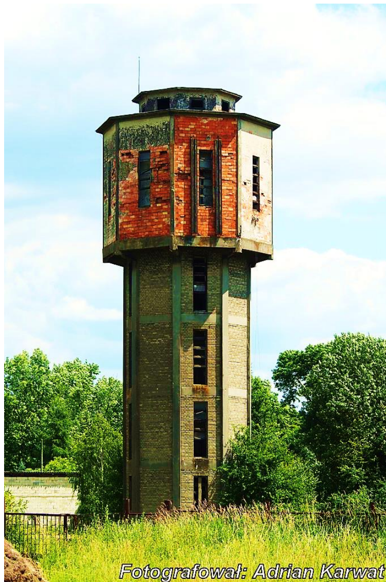
Water tower (for steam locomotives)
