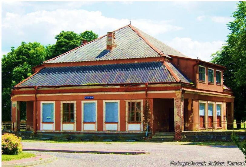
Railroad statkion building
